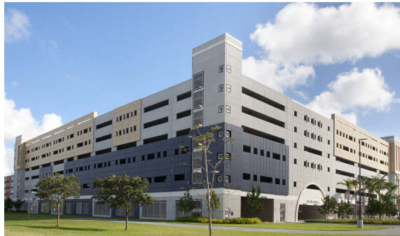
Figure 1: Parking garage with approx. 2,000 parking spaces
