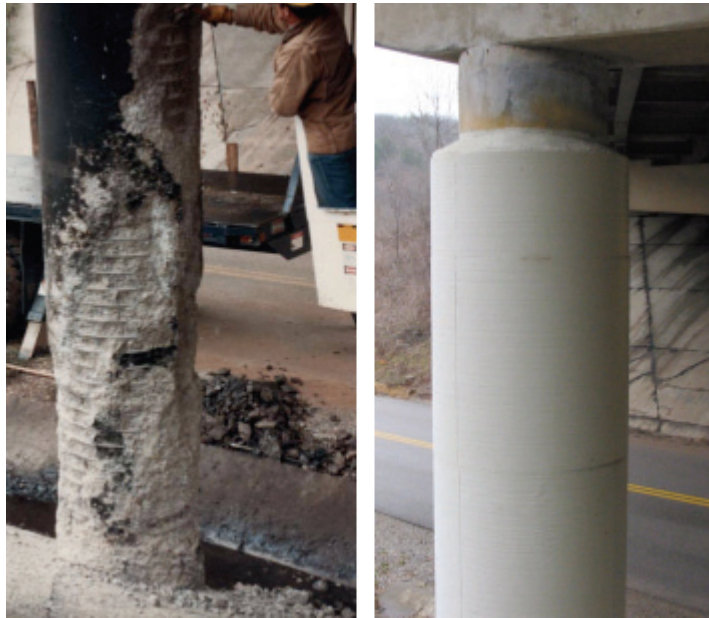
Before and after composite wrapping.
