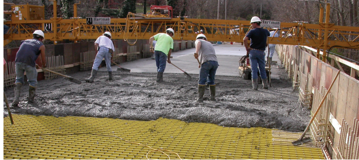
Construction workers walking on GRIDFORM reinforcement while placing concrete GRIDFORM panels.
