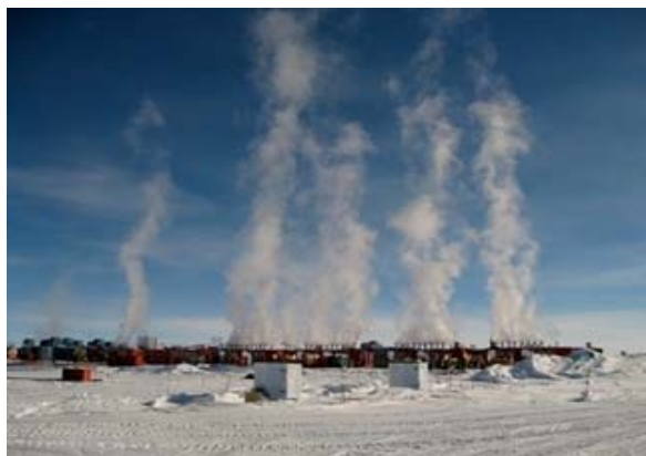
Steam rising from the IceCube heating plant. Credit: Jim Haugen, University of Wisconsin-Madison, 2008.
