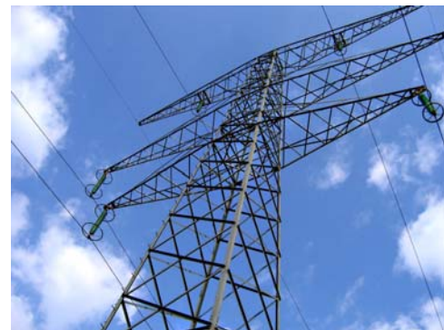
TCIP researchers work to provide end-to-end secure and real-time power grid monitoring and control. Credit: http://commons.wikimedia.org/wiki/File:Ligne_haute-tension.jpg .
