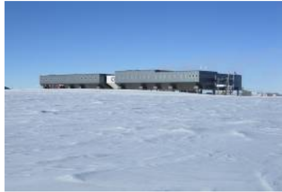
South Pole Elevated Station, which exceeded new federal standards for energy efficiency even in the harsh environment of Antarctica. Credit: Jerry Marty.
