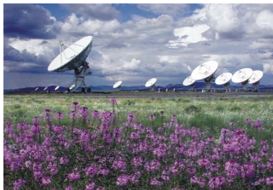
The Very Large Array (VLA) telescope, located about 80 km west of Socorro, NM, is composed of 27 individual antennas arranged in a "Y" pattern. In their closest configuration (about 1 km wide), the VLA is able to image large portions of the sky. In its largest configuration (about 36 km wide) the VLA is able to home in on the fine details of astronomical objects. Credit: NRAO/AUI and Kelly Gatlin, Patricia Smiley.
