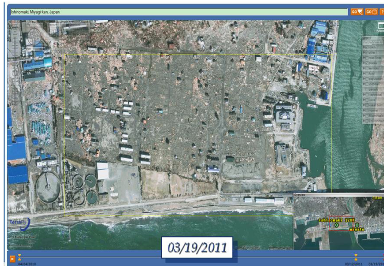
Figure 7. Ishinomaki, Japan, 8 days after the earthquakes and tsunami of March 11th, 2011
